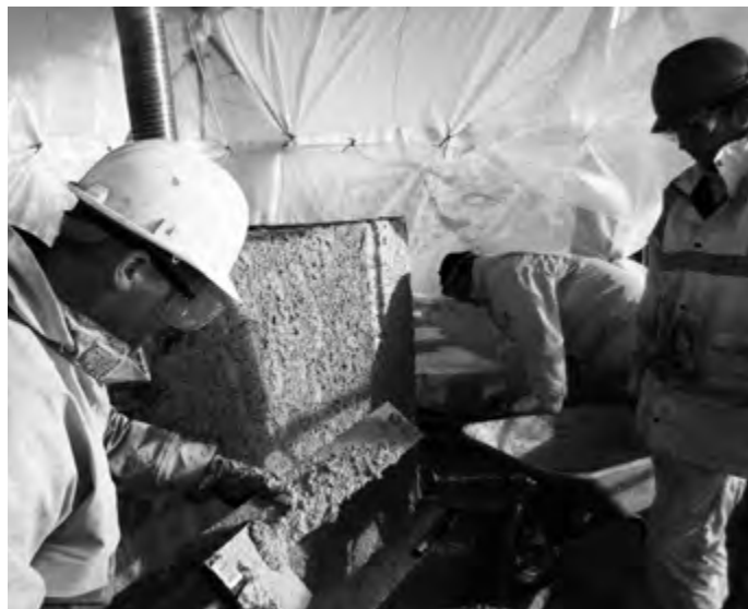
Harling in progress at the Old Haa, Sand
