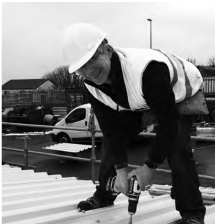
Work underway on the Scalloway Museum extension.
