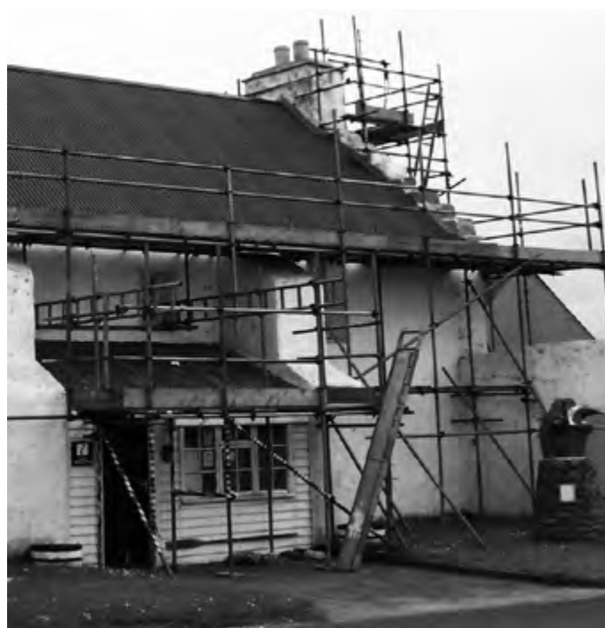
Roof repairs at the Old Haa, Burravoe
